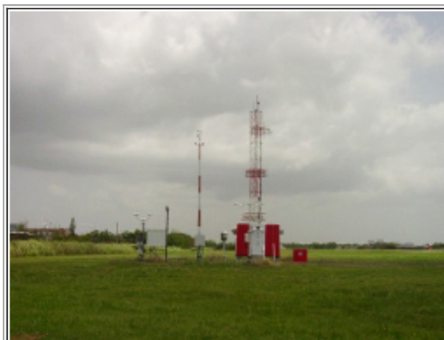
The Automated Airport Weather Station (ASOS) at the Luis Muñoz Marín International Airport in San Juan (looking West).
